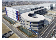
Misato 1 Logistics Centre
